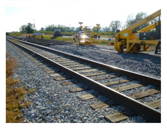
The second major rail construction project is the expansion of the South Rail Loop. The initial, single, rail loop track constructed in 2009, will now have two additional adjacent tracks to meet the growing rail needs at the Harbor. Over 15,185 feet of rail will be constructed in this project, allowing additional train capacity.
